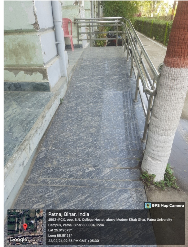
RAMP for Main Building
