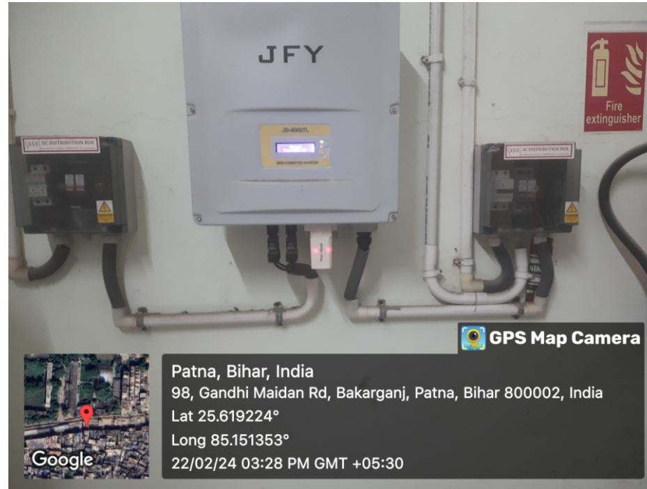
Inverter and AC & DC box of solar power plant
