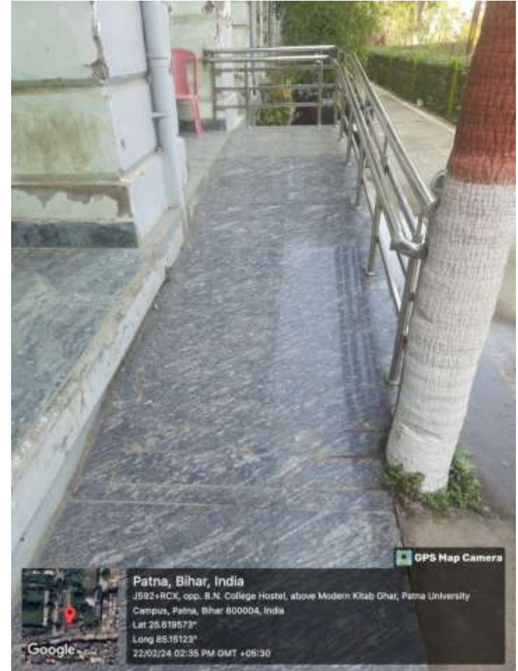
RAMP for Main Building
