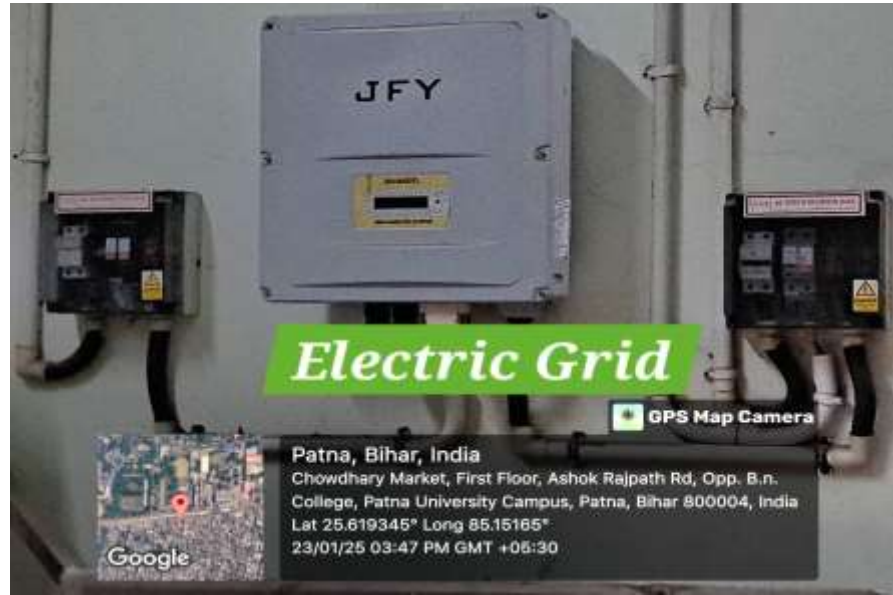
Inverter and AC & DC box of solar power plant
